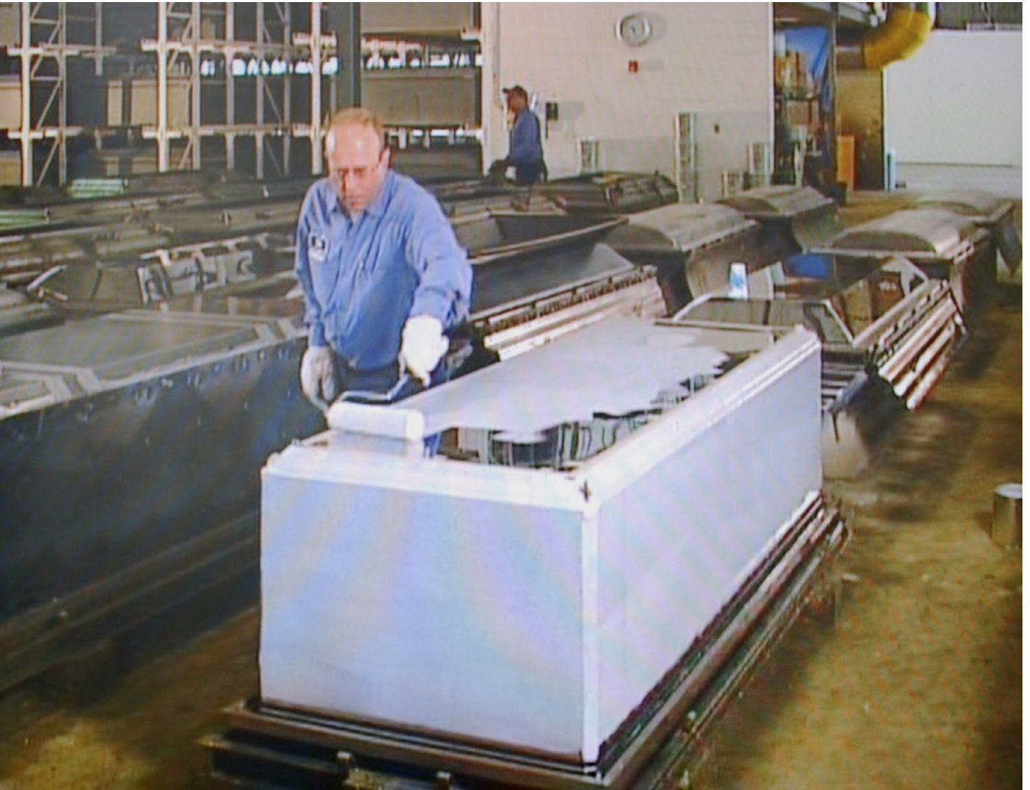
The pieces of the stainless steel liner are assembled on the mold, then coated with an adhesive for bonding with the high impact plastic liner. Note: the vault is manufactured upside-down and from inside out
